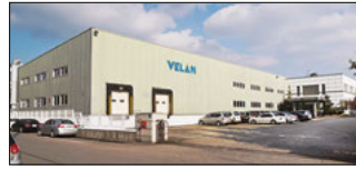
Ansan City, South Korea Velan Ltd., Plant 2
