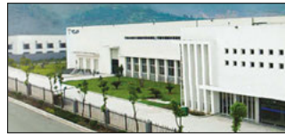
Suzhou, China Velan Valve (Suzhou) Co., Ltd.
