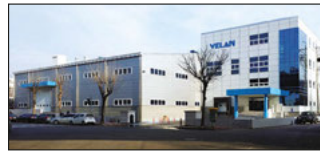
Ansan City, South Korea Velan Ltd., Plant 1
