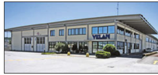
Lucca, Italy Velan ABV S.r.l., Plant 2
