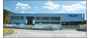
Lucca, Italy Velan ABV S.r.l., Plant 1
