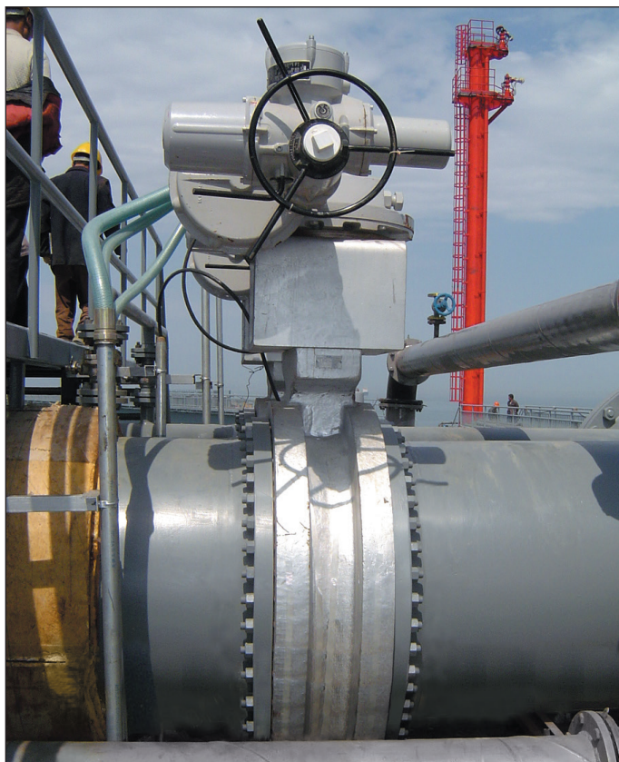
A large Torqseal™ triple offset valve used for crude oil service in the Dalian Seaport (China).
