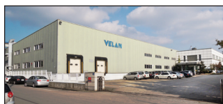
Ansan City, South Korea Velan Ltd., Plant 2
