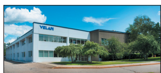
Williston, VT, U.S.A. Velan Valve Corp.
