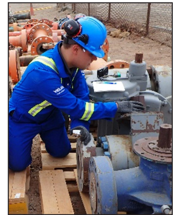
On-site service for Velan valves.
