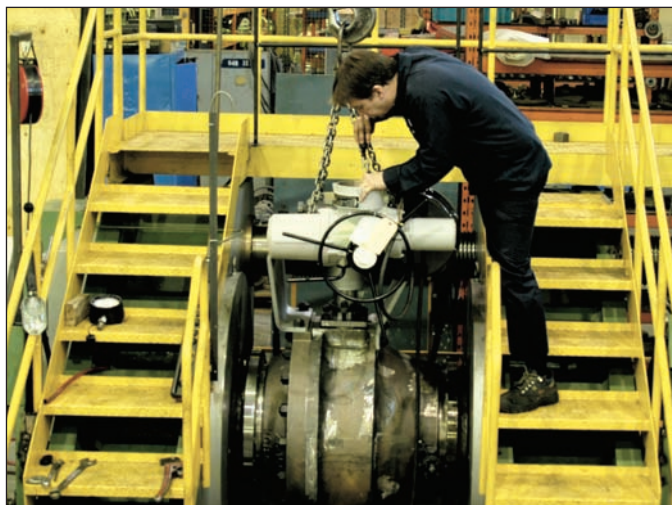
An actuator is installed on a metal-seated ball valve before hydrotesting.
