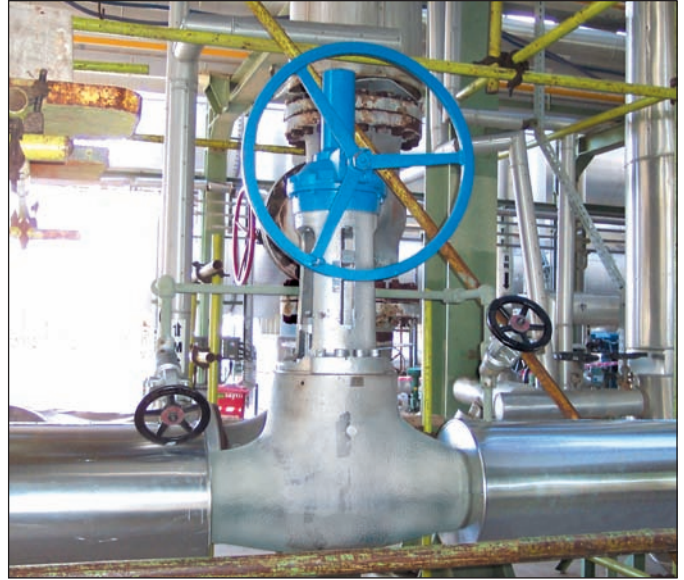
A 10" (250 mm) pressure seal valve at a refinery in Brazil.
