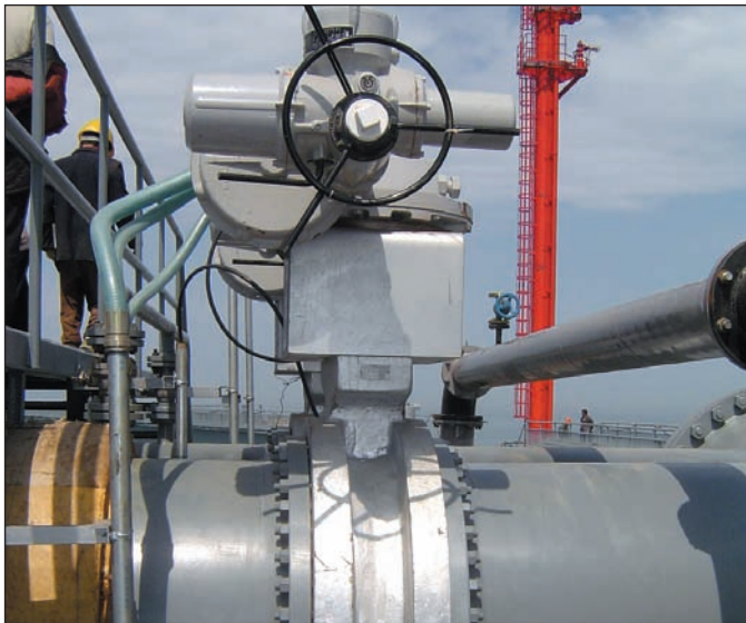
A large Torqseal™ triple-offset butterfly valve used for crude oil service in Dalian Seaport (China).
