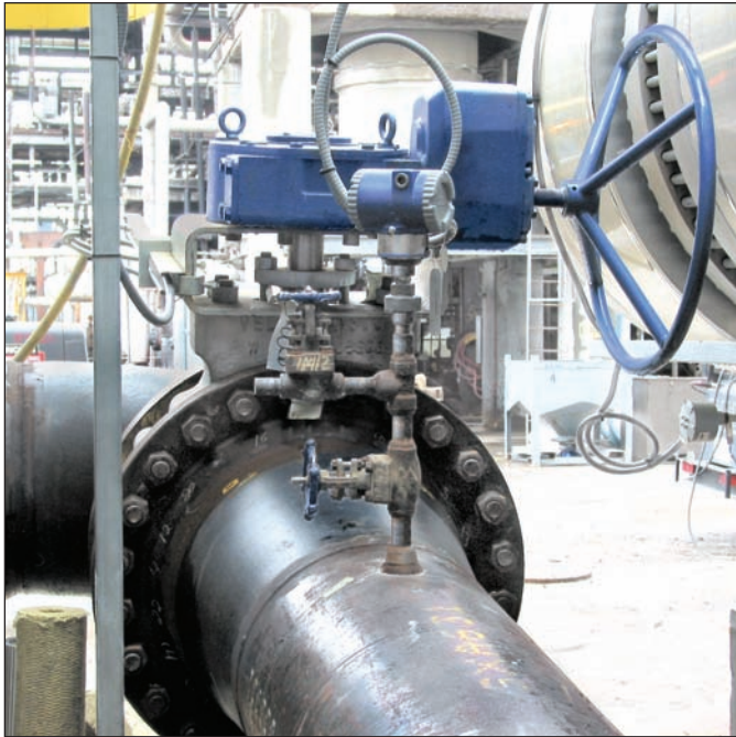
20" (500 mm) class 150 Torqseal™ valve on cooling water isolation to the heat exchanger.
