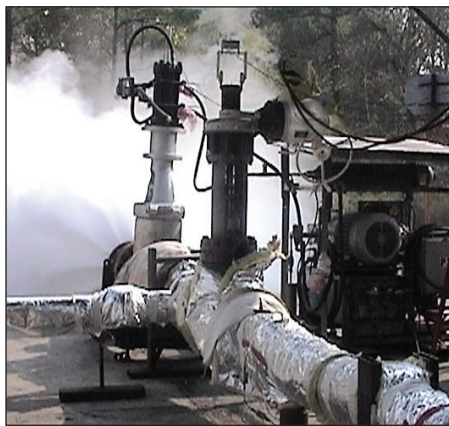
Line break testing (blowdown) (1)
