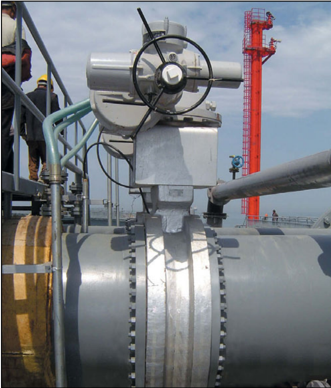
A large Torqseal™ triple-offset valve used for crude oil service in the Dalian Seaport (China).
