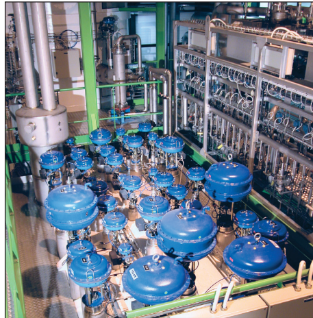
Some of the 2,500 Velan cryogenic valves for liquid helium installed in the Large Hadron Collider (LHC) at CERN.
