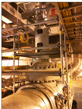
Gasket replacement on a 30" Velan bolted bonnet gate valve
