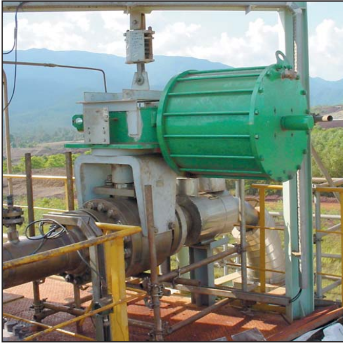
Securaseal severe service ball valve with pneumatic actuator.
