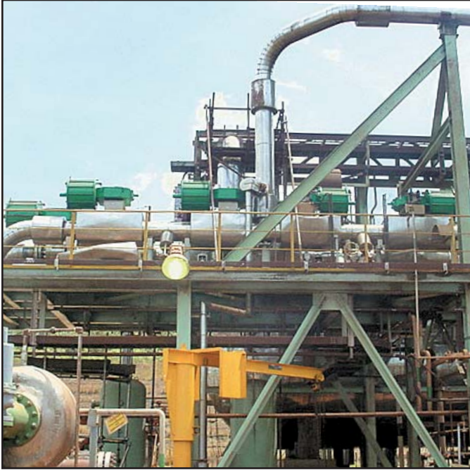
Velan Securaseal severe service ball valves for mineral extraction in service.
