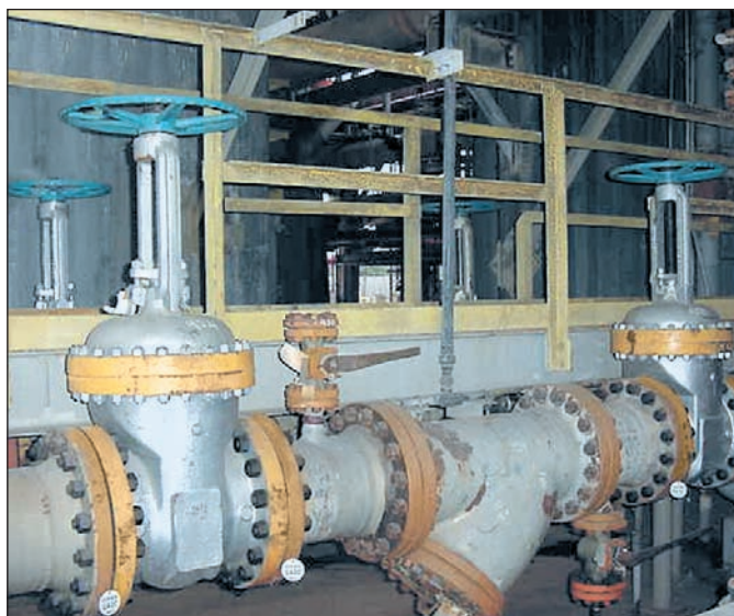
Two HF acid 12" (300 mm) class 300 gate valves installed at ExxonMobil.
