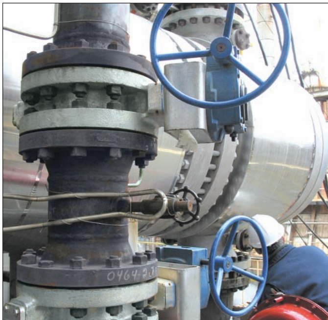
A double block and bleed setup using a 12" (300 mm) class 300 347 stainless steel Torqseal™ valve on hydrogen service at 500 psi/900°F (34.5 bar/482°C).
