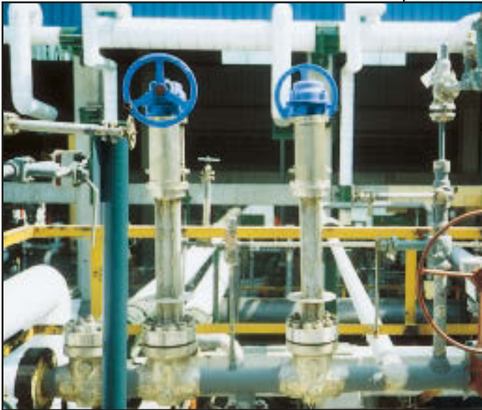
Gate Valves, 1/4–48" ASME Classes 150–2500, Forged 1/4–24", Cast 2–48"
