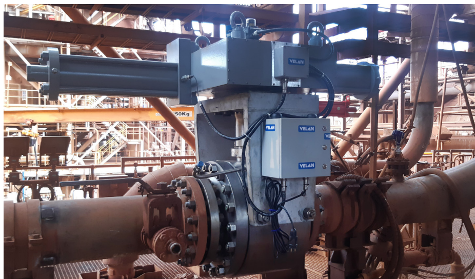
For a mining end user, the Velan Online Monitoring System is combined with a Velan NPS 12 Class 300 severe service valve and the Velan Cable Drive actuator to monitor the operating torque.
